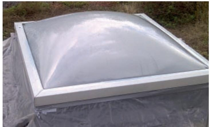
**When coating skylight domes with a frame, please remember to also coat the upper surface of the frame.** This means the adhesive masking tape must be fitted below the frame. Only remove the masking tape once the material is sufficiently dry to prevent any "runs" or "drips".
