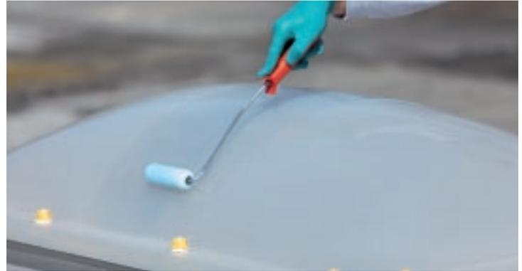
The liquid material may "run" and "drip" depending on the shape and positioning of the skylight dome. Therefore, brush over the wet material several times after a few minutes, always working from bottom to top. This guarantees an even layer thickness over the entire skylight dome.
