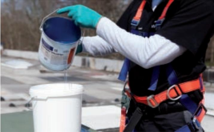
It is then advisable to weigh the material individually for each step based on the square metre size of the skylight dome (**400 g/m<sup>2</sup>/work step**).
