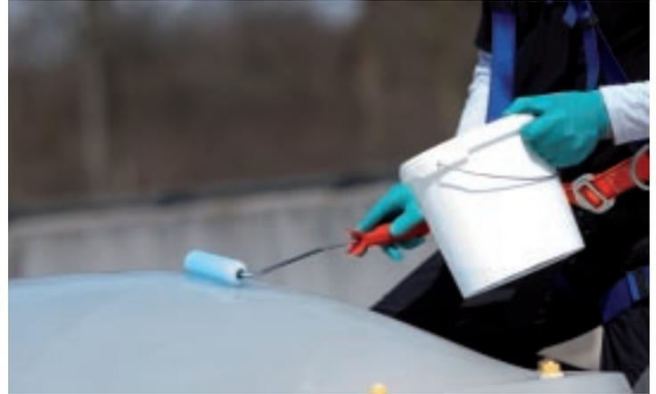
The material is either gradually poured onto the skylight dome or applied directly from the container. Distribute the material using a foam roller in a criss-cross fashion.
