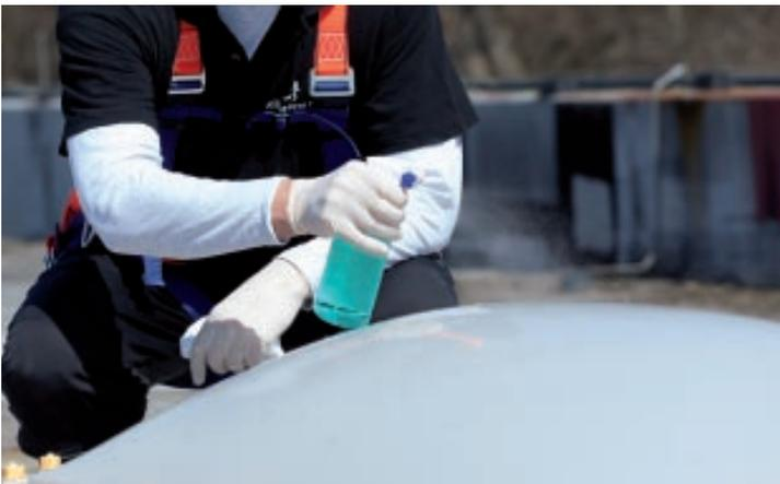
**New and unweathered skylight domes** must be cleaned carefully using a lint-free cloth and KEMPERTEC® FALLSTOP Cleaner. Only start coating the skylight dome once the cleaner has fully evaporated (approx. 15 minutes).
