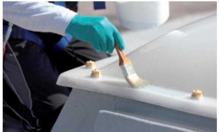
The lower frame/edge of the skylight dome is coated using a foam roller or brush. Brush any material that has run down the frame/edge upwards
