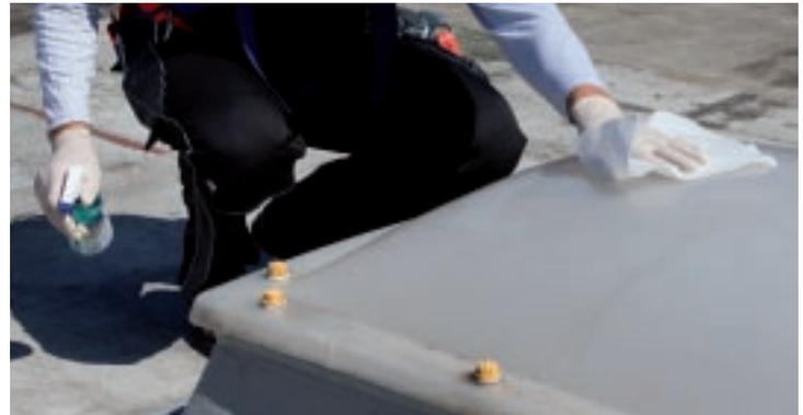
**Old and weathered skylight domes** must be cleaned carefully using a mop and water prior to application. Then thoroughly clean the skylight dome using a lint-free cloth and KEMPERTEC® FALLSTOP Cleaner in order to remove any loose particles and substances from the substrate that may reduce adhesion. You can start coating the skylight dome after approx. 15 minutes once the cleaner has fully evaporated.
