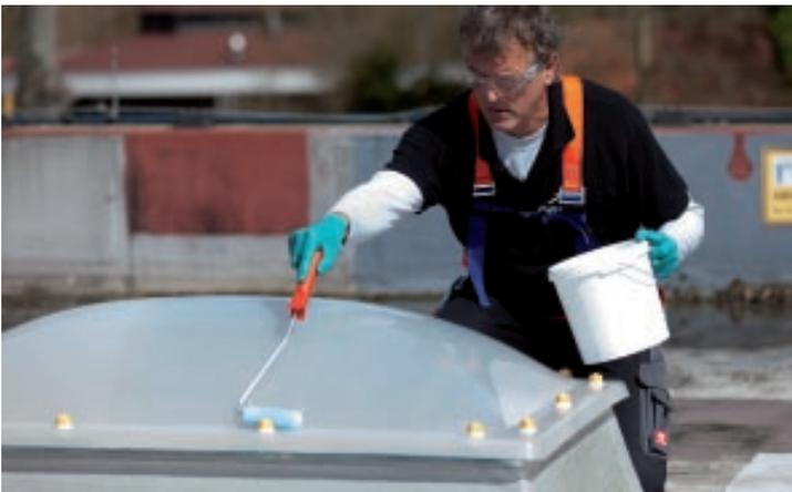
The material must be applied evenly and free of bubbles horizontally and vertically. **Practical tip:** When applying the material, the foam roller should work silently, as roller noises are an indication of insufficient material application.
